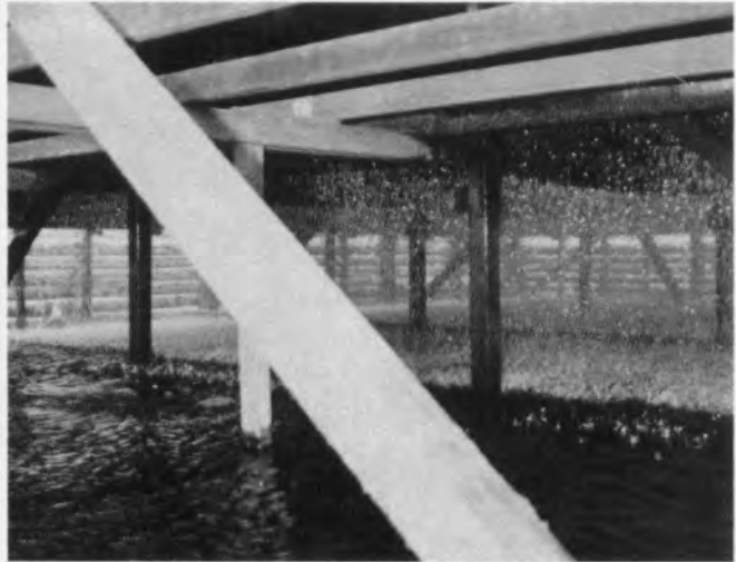
Proper nozzle selection ... means uniform coverage and more efficient cooling.
