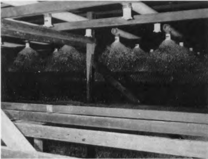
Proper nozzle selection ... means uniform coverage and more efficient cooling.
