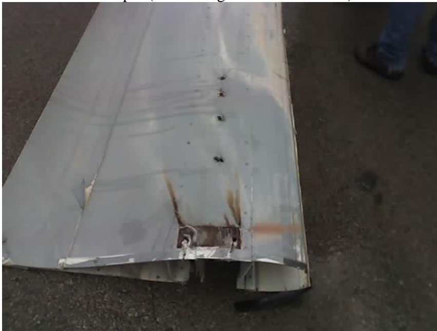
Photo of failed blade which has separated from the spar and the hub.
